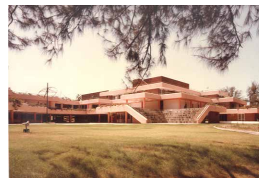
Photo courtesy: Charles Correa Foundation ; 1985, River fronting (rear) view of Kala Academy, Goa.
